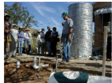
Figure 6 Steel Culvert Cistern
