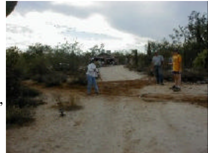
Figure 13 Constructing a Swale
