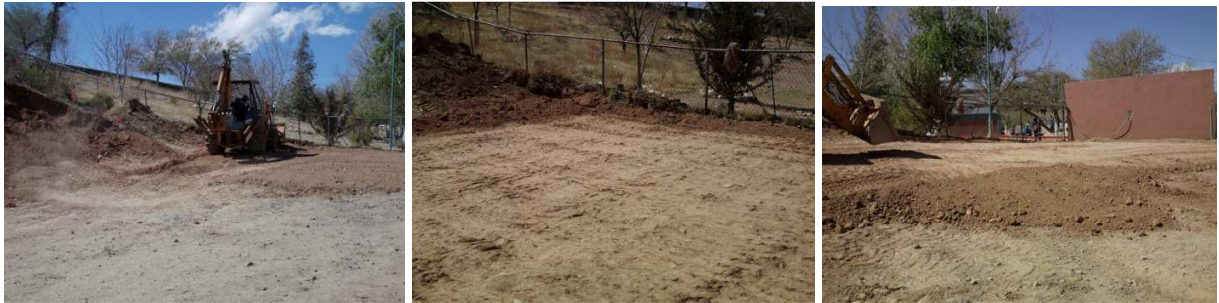
Figure 3.2.a. Initial site preparation
