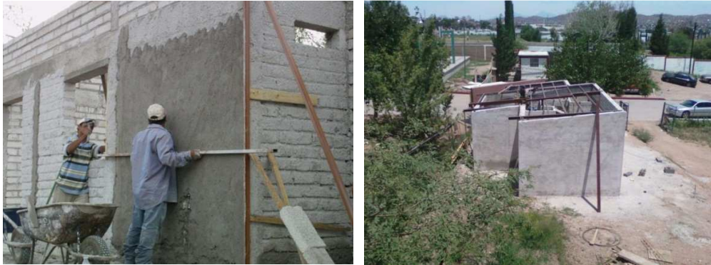
Figure 3.2.d. Applying regular cement plaster to exterior walls
