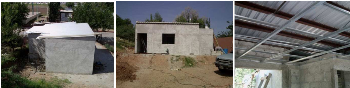
Figure 3.2.e. Installing the roof
