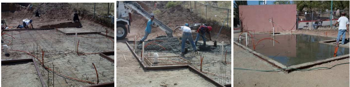
Figure 3.2.b. Laying the foundation
