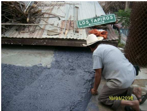
Figure 4.5. Local entrepreneur learning to apply fibrous concrete insulation to an existing roof
