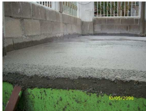
Figure 4.5. Local entrepreneur learning to apply fibrous concrete insulation to an existing roof
