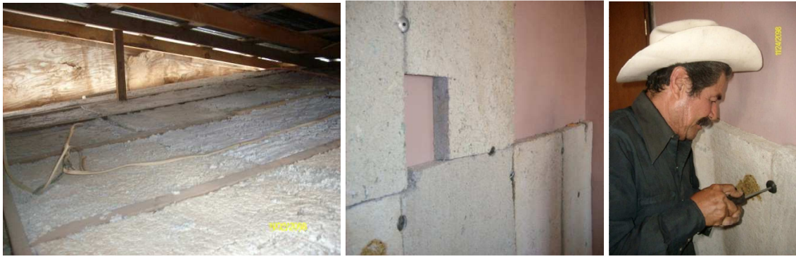
Figure 2.7. Panels made of fibrous concrete in a 1:1 ratio of paper to cement
