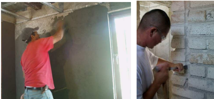
Figure 3.2.f. Applying fibrous concrete stucco to interior walls
