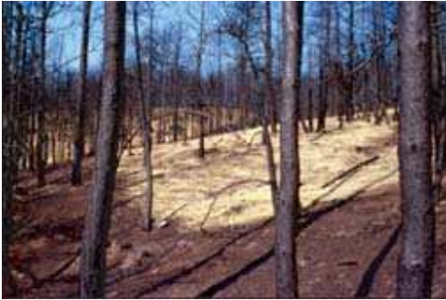
Spread straw over seeded area to prevent erosion
