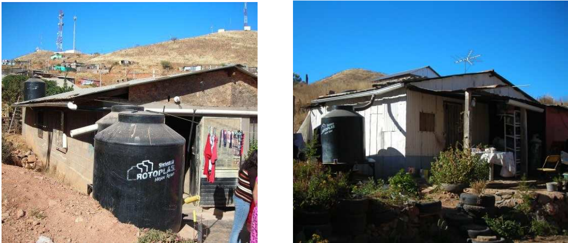
Figure 4. Photos of Active Household Water Harvesting Systems
